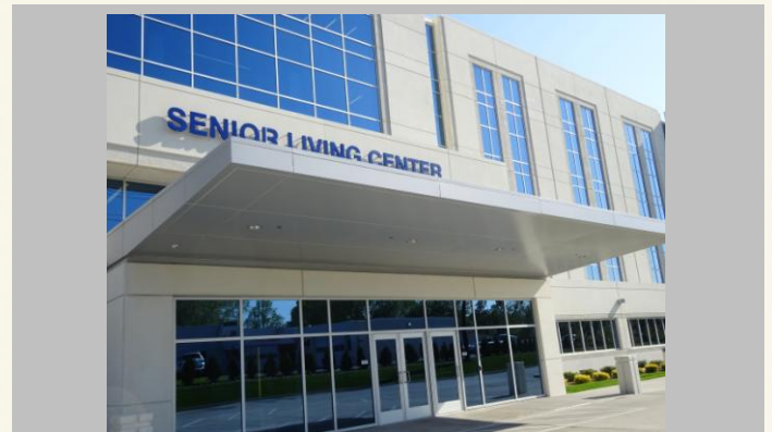
The Senior Living Center (Erie, PA) consisted of metal screen wall panels, TPO roof system, aluminum composite wall, and soffit panels.
